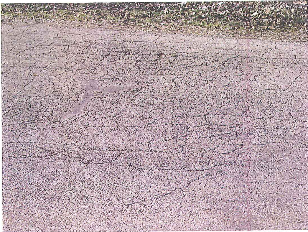
Picture 3 – Pavement Segment 305 (3100 Memorial Shoreway)
