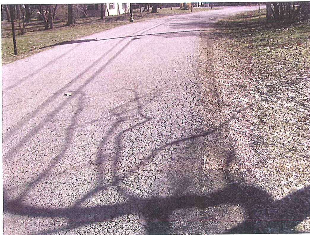
Picture 4 – Pavement Segment 306 (3116 Memorial Shoreway)
