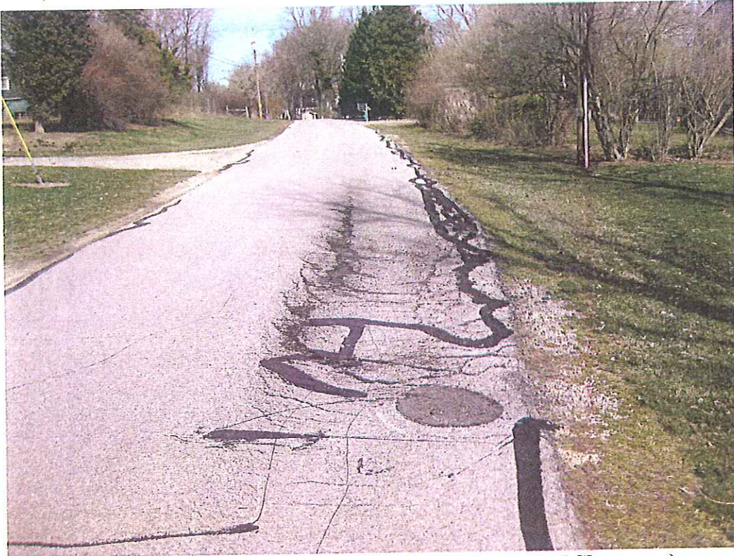
Picture 33 – Pavement Segment 366 (4430 Memorial Shoreway)
