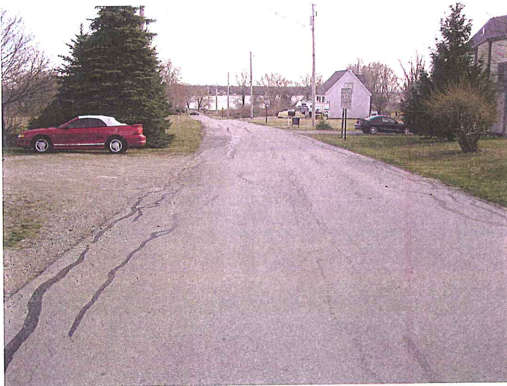
Picture 40 – Pavement Segment 101 (Gaydos Drive south from Bayshore)
