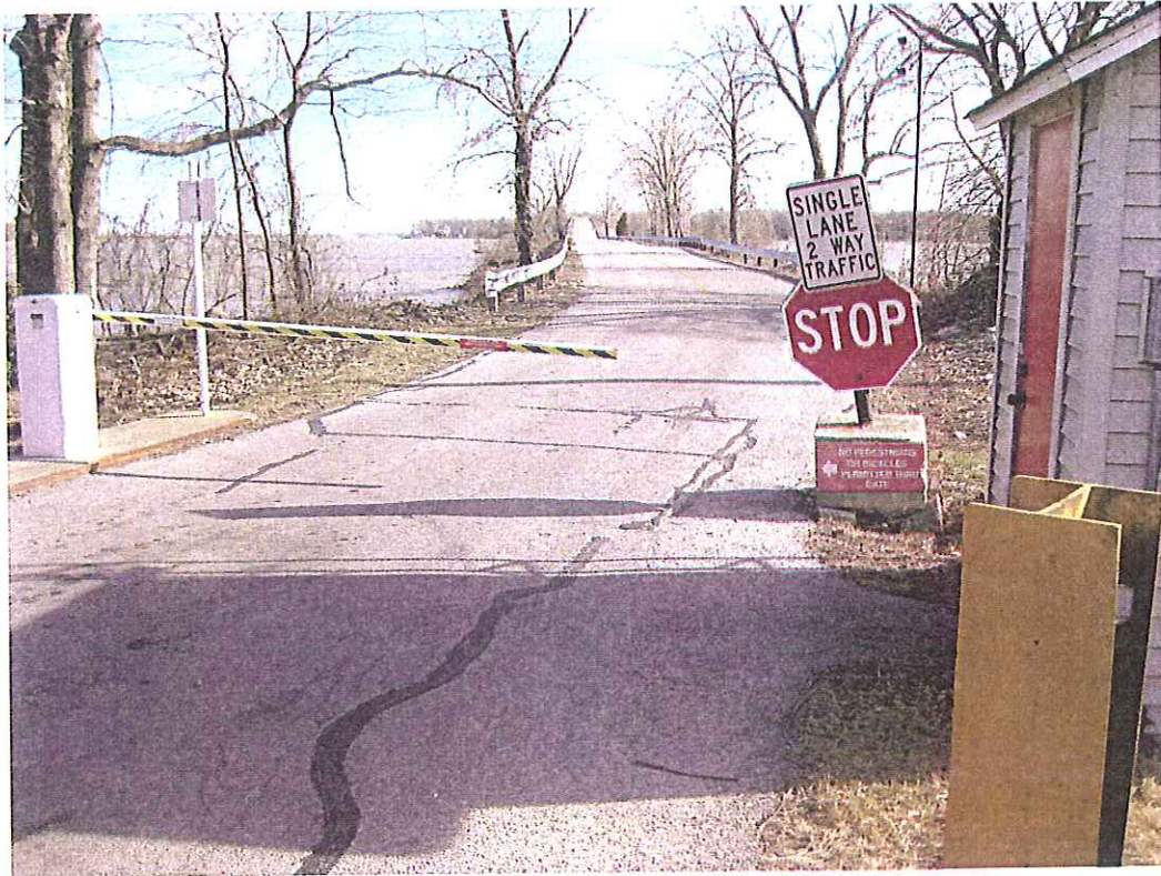
Picture 39 – Pavement Segment 103 (Gaydos Drive south to Causeway)
