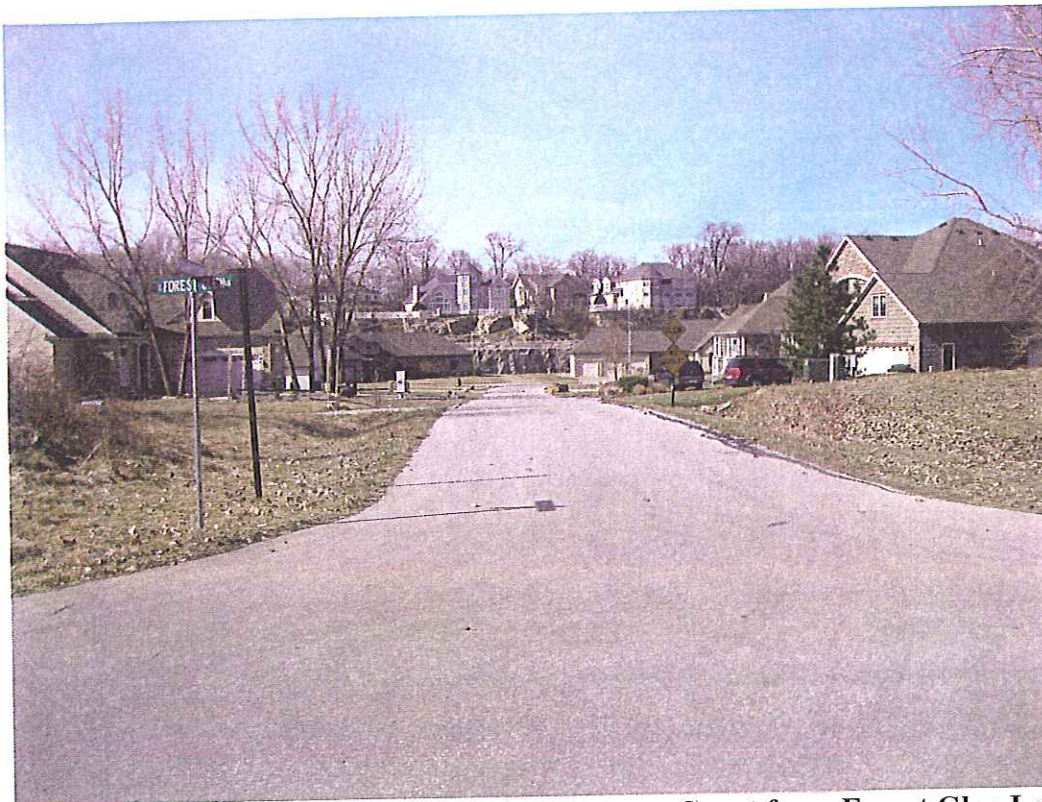
Picture 36 – Pavement Segment 801 (Quarry Stone Court from Forest Glen Lane)
