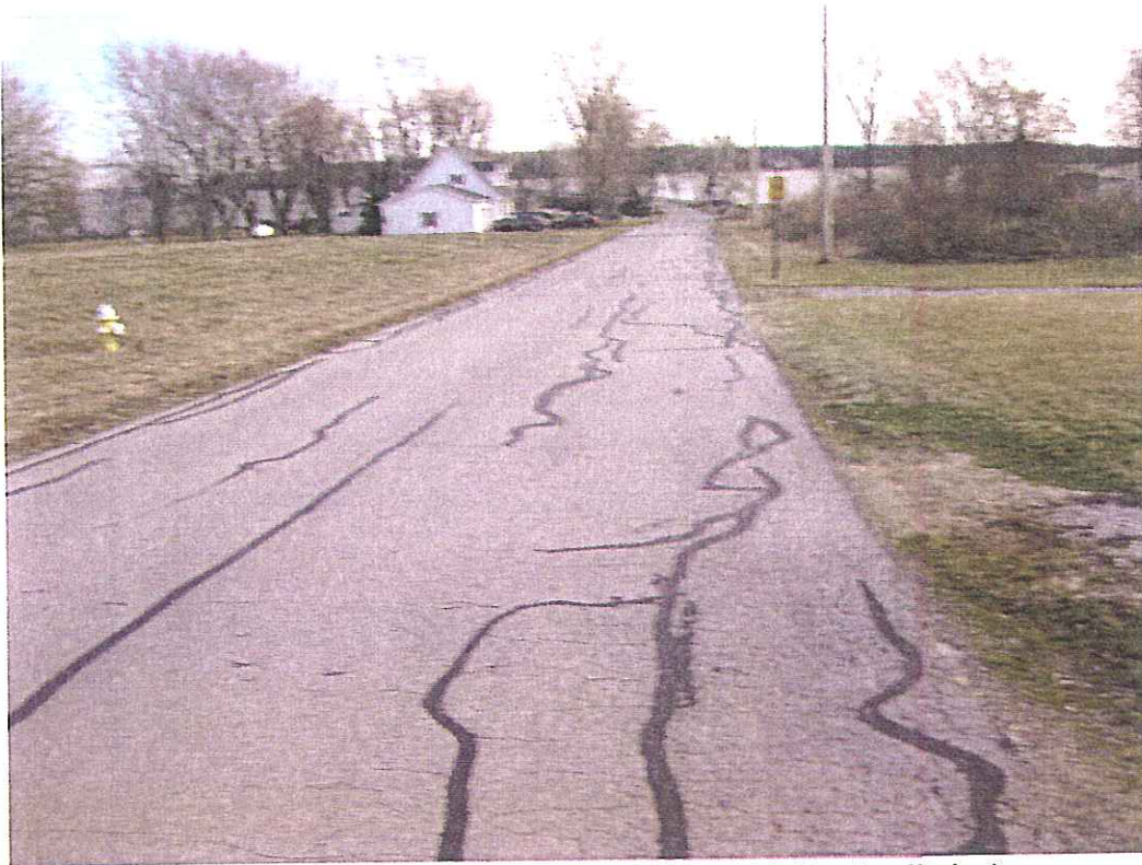
Picture 43 – Pavement Segment 102 (8076 Gaydos Drive)
