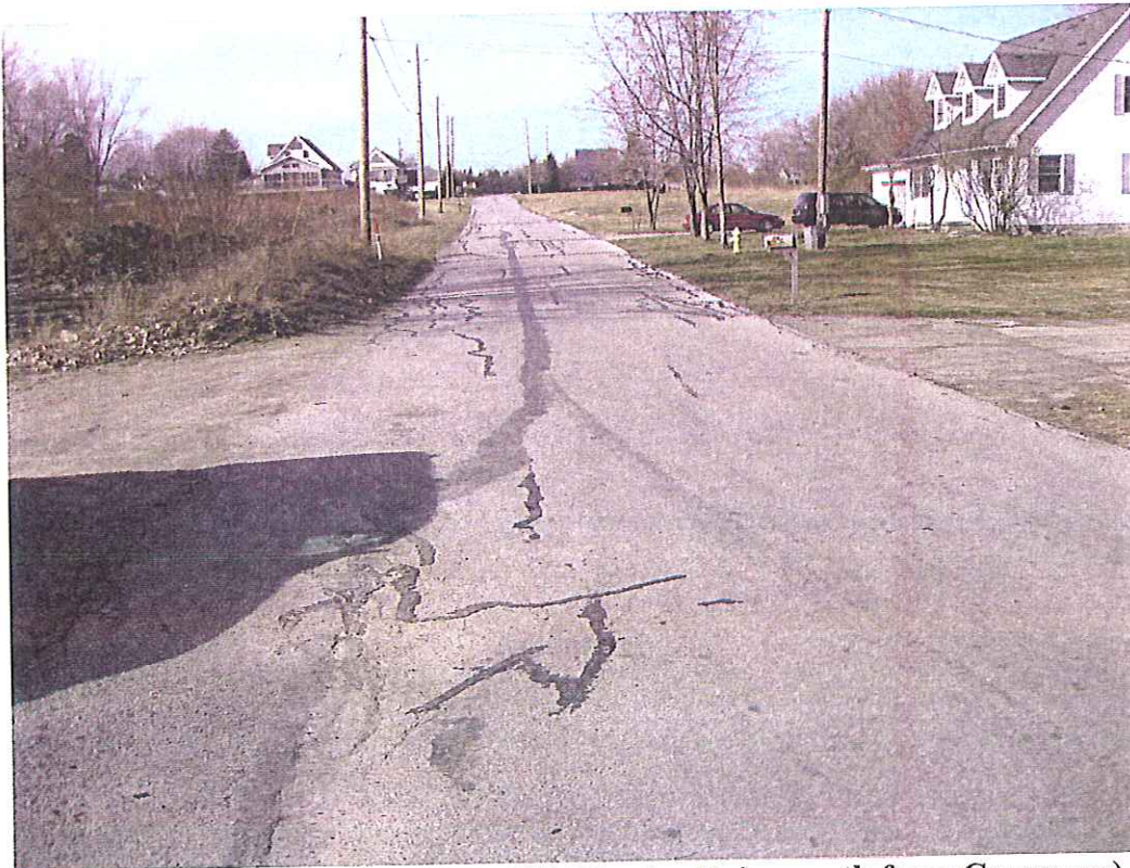
Picture 38 – Pavement Segment 103 (Gaydos Drive north from Causeway)
