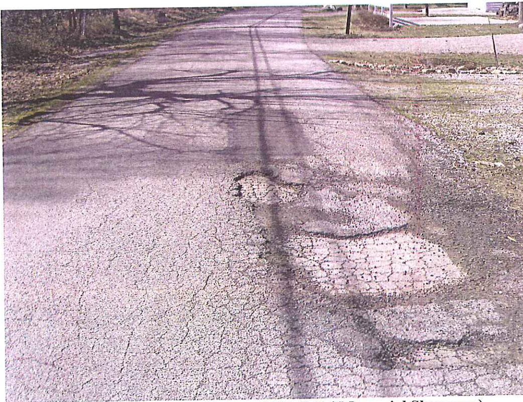
Picture 14 – Pavement Segment 323 (3416 Memorial Shoreway)
