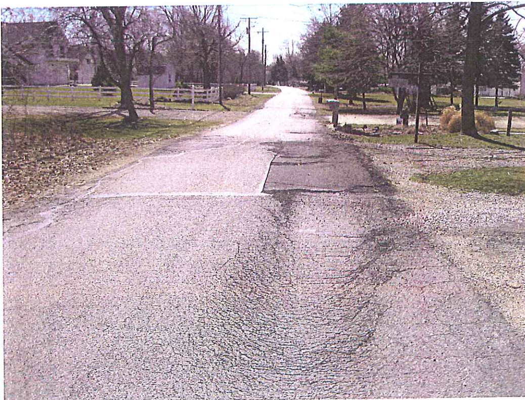
Picture 24 – Pavement Segment 347 (3972 Memorial Shoreway)
