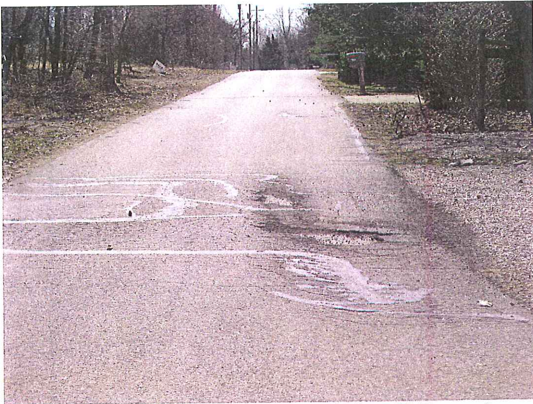
Picture 23 – Pavement Segment 344 (3914 Memorial Shoreway)
